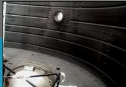
2. RTT Sealant spray applied to entire area
