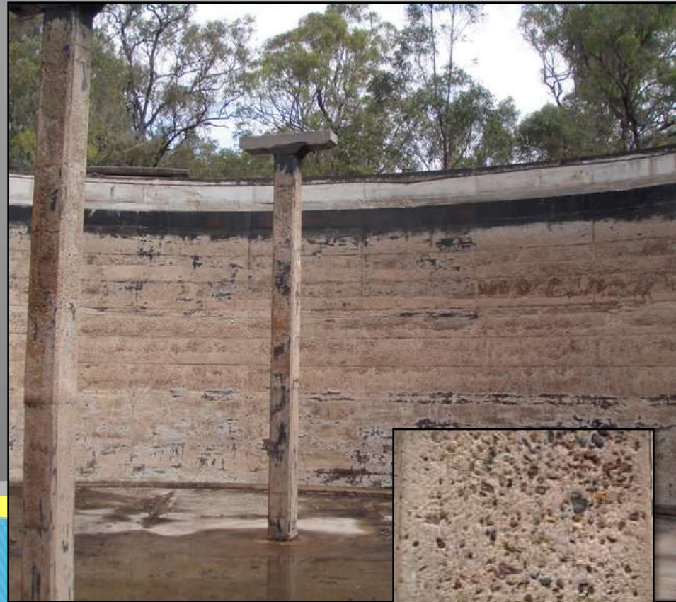
Pressure washed back to bare concrete
