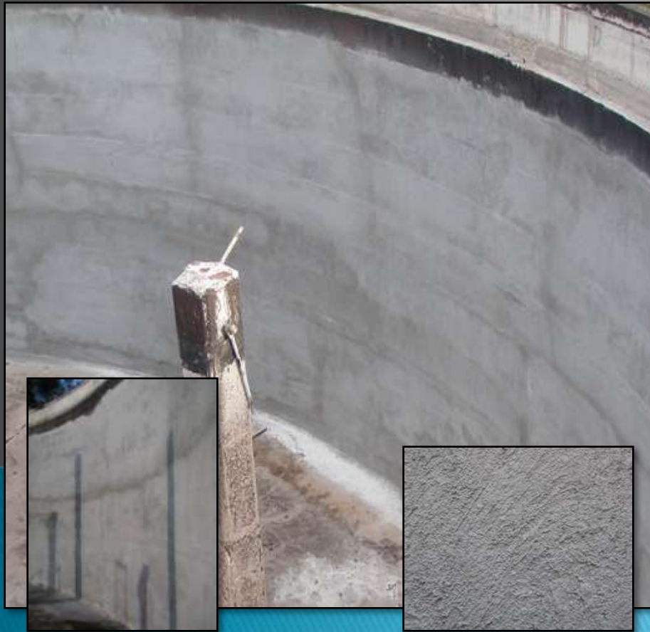
Walls rendered to fill holes and cracks
