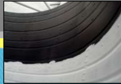
3. Coloured top coat applied to RTT Sealant
