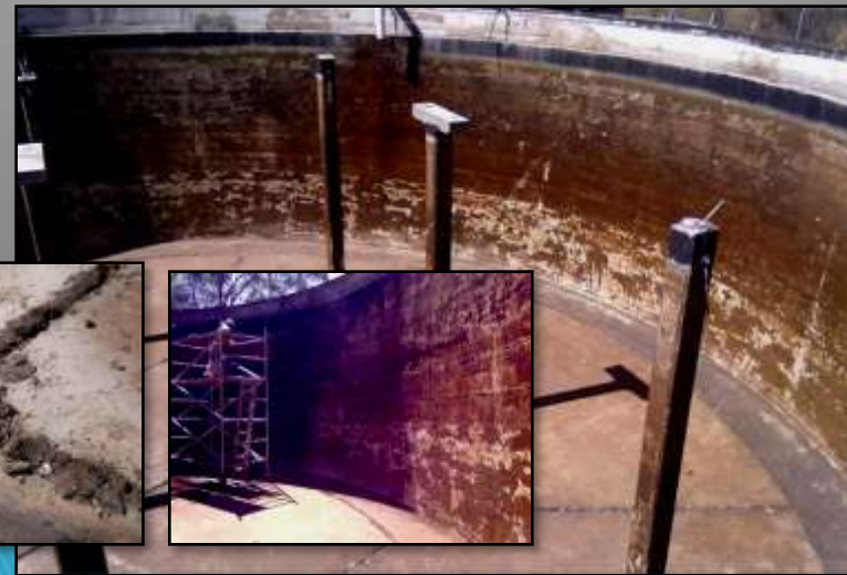
Floor joints and wall before cleaning
