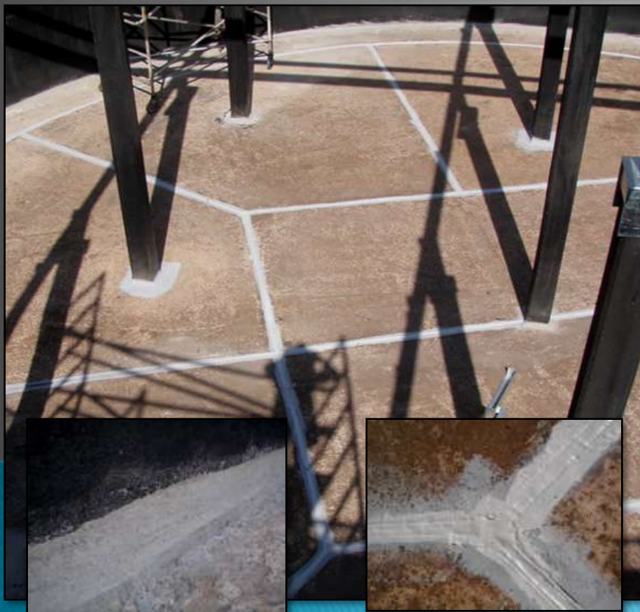
Wall floor joint coved and expansion joints filled
