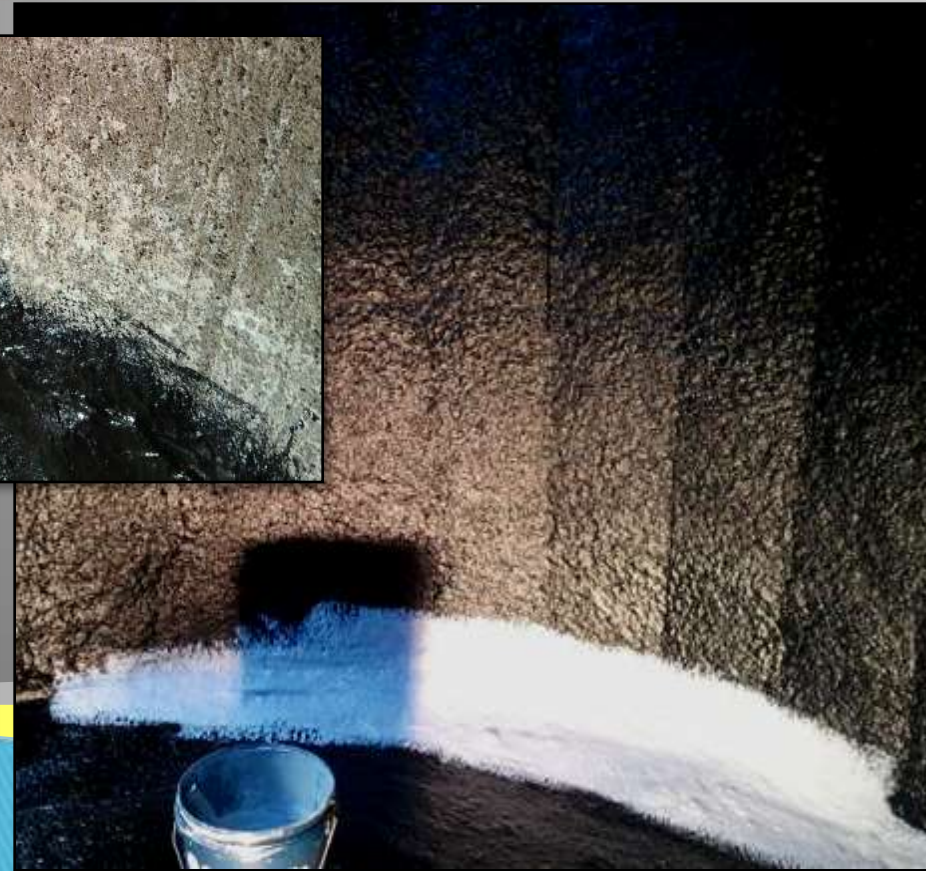
4. RTT Sealant coated with coloured reinforcing top coat
