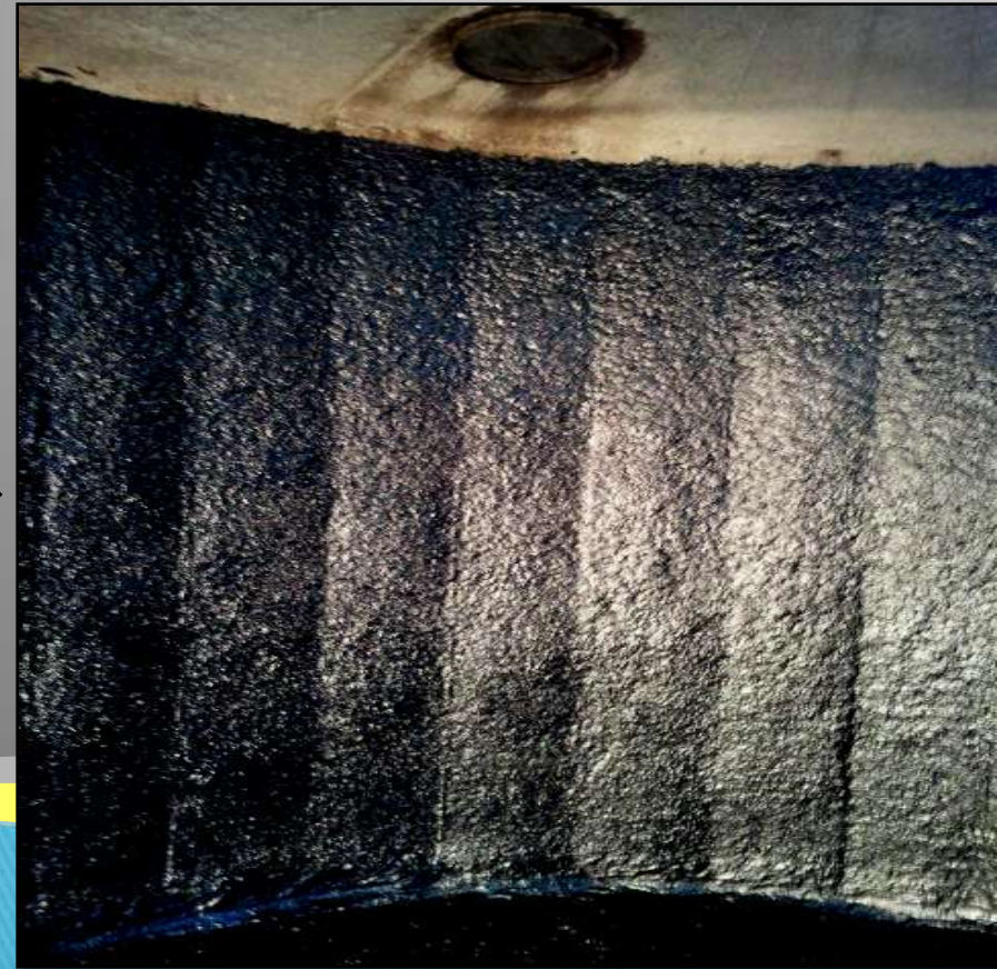
2. RTT Sealant applied to surface
