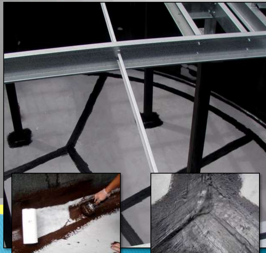
Floor sealed and joints and corners reinforced
