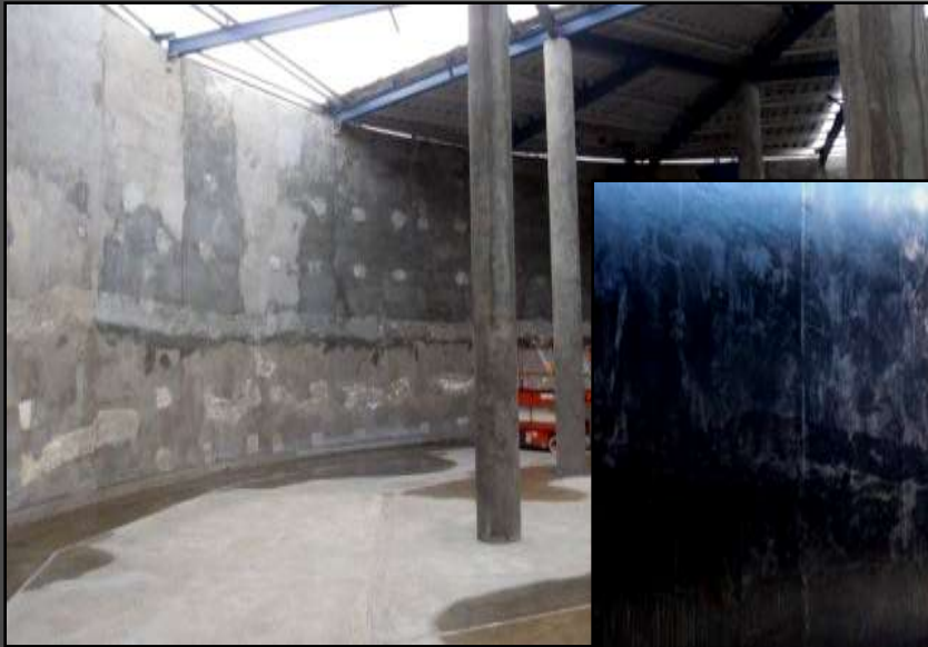
1. Bare concrete tank wall
