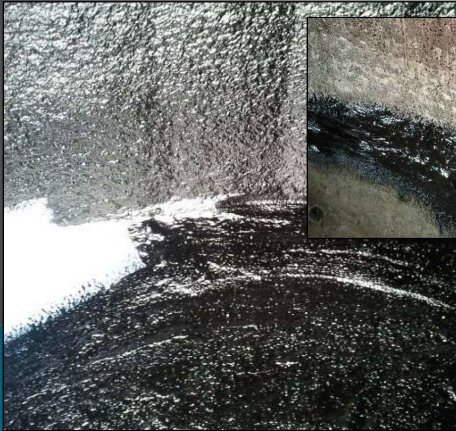
3. Corners reinforced and top coat applied
