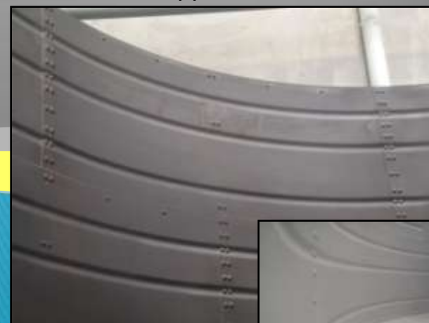
RTT Sealant + Top coat spray applied
