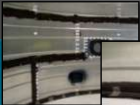
1. RTT Sealant applied to joints and corners
